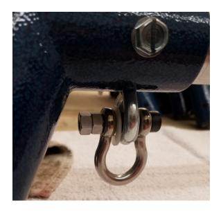
Both views below show the chain connectors installed. Make sure the spring clips have closed properly. The position shown to the left is for linear movement of the swing. If rotation is desired, place both connectors in the single point connection. This is shown in the view to the right.
